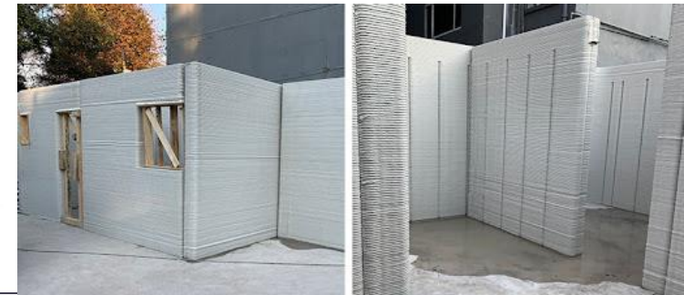
A model of a RDP house, UJ revealed it was built in a day using 3D printing
